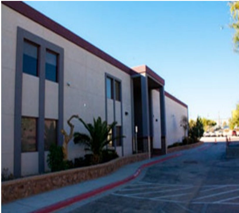
Middle School Building
